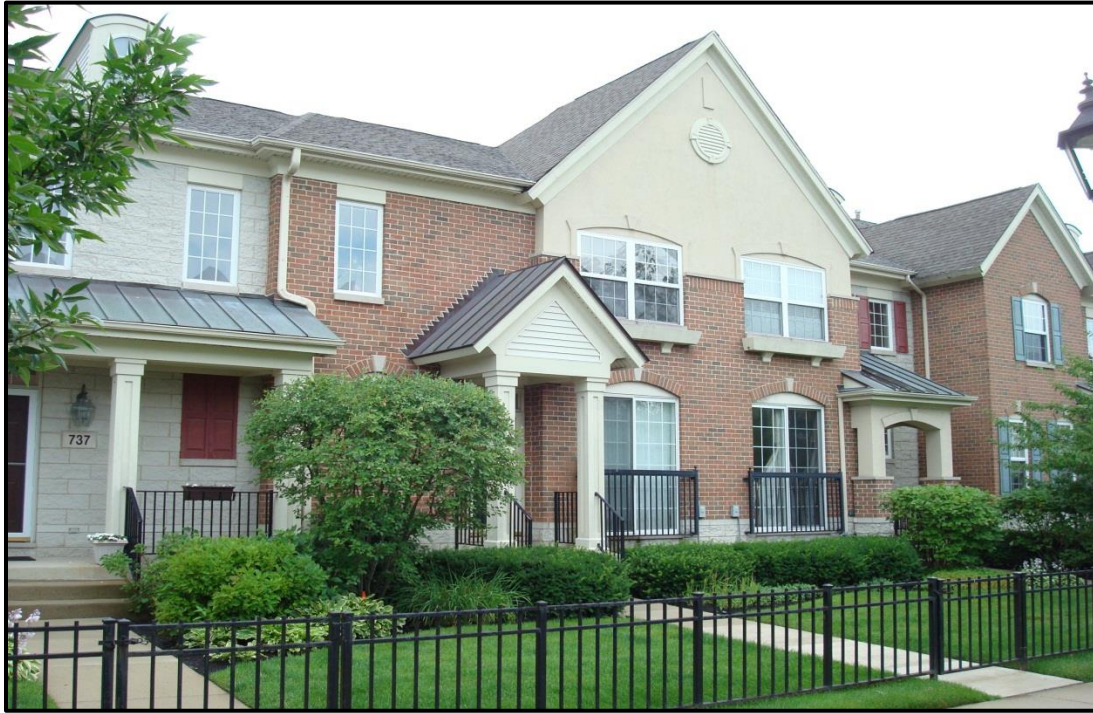
Photo 14. These town houses in Deerfield are Auto-urban residential as they likely require an automobile for a majority of their day to day services.
