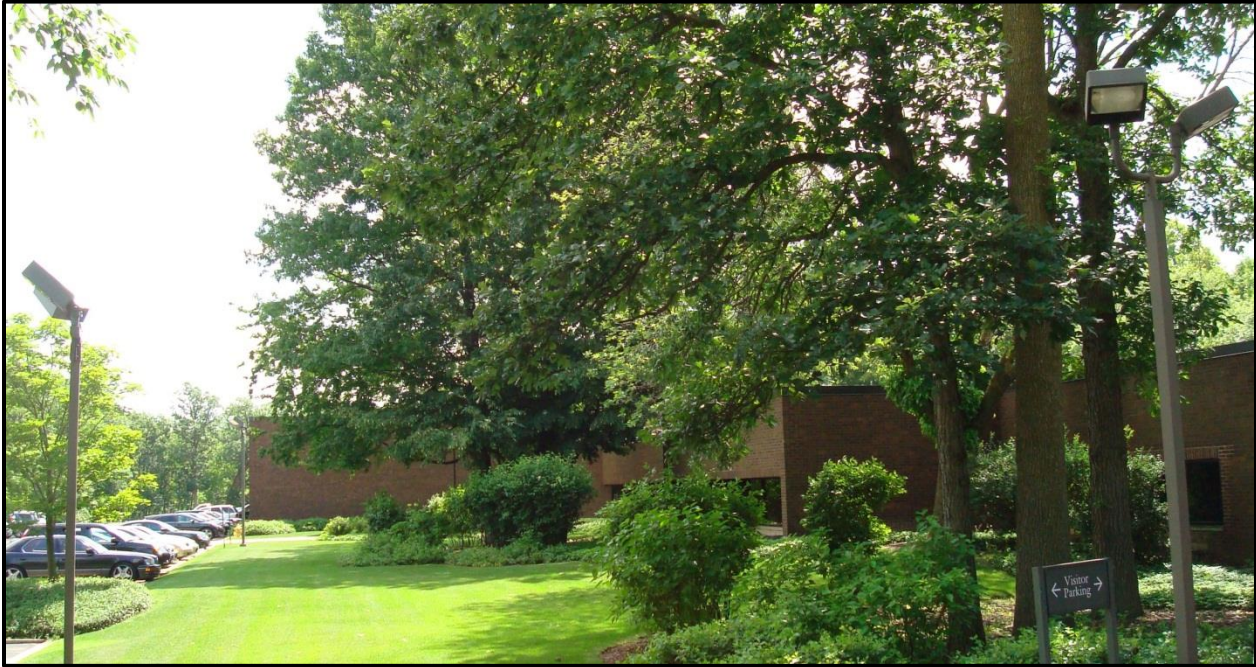
Photo 35. Terlato Wine Group preserved trees and used ivy on the walls to soften the building's impact.
